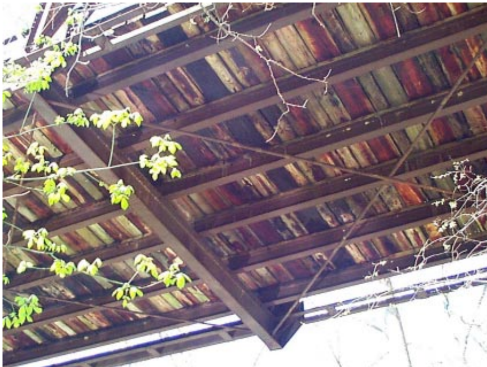
UNDERSIDE OF TRUSS BRIDGE
