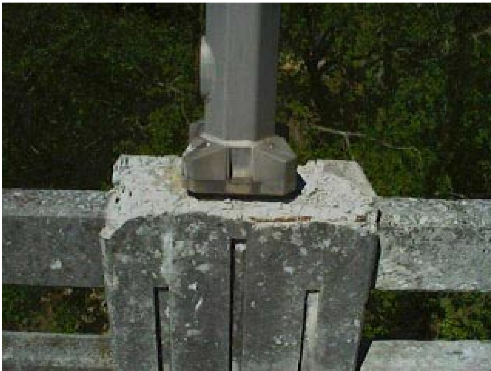
CONCRETE BRIDGE RAIL AND METAL POST
