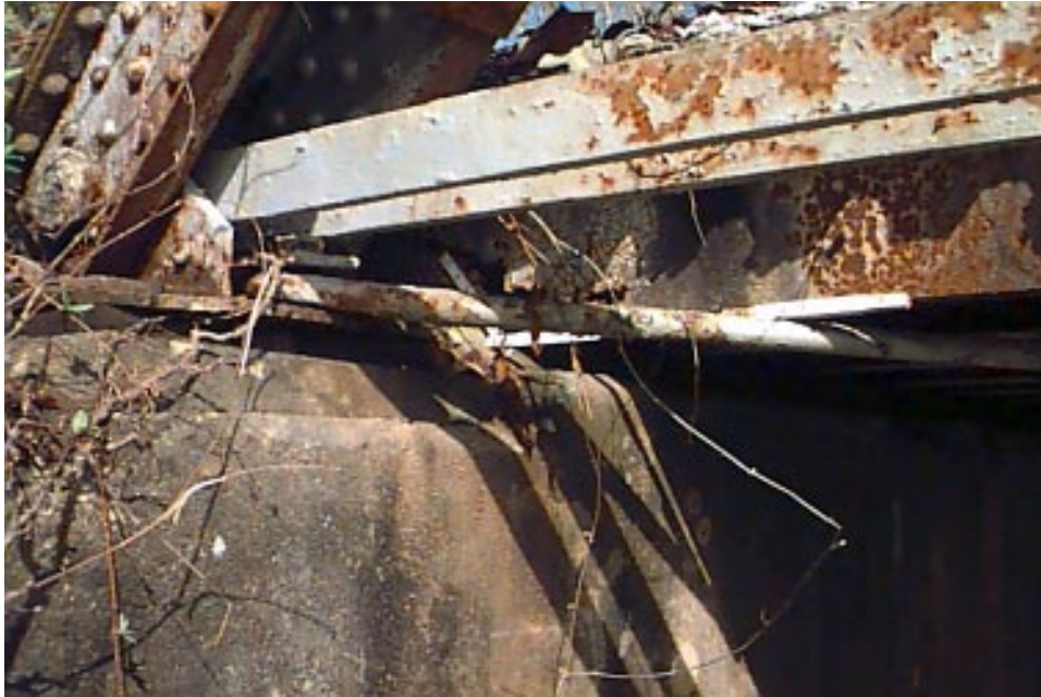
LOWER CHORD OF STEEL TRUSS
