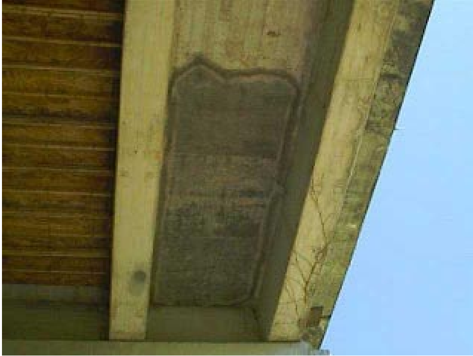
PATCHED AREA IN CONCRETE DECK
