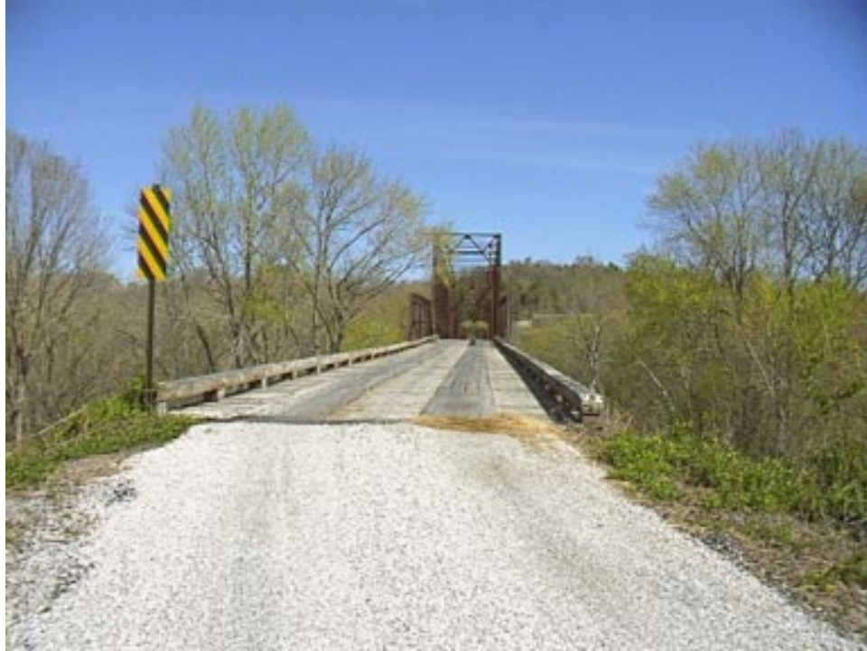
ROADWAY APPROACH TO STEEL TRUSS BRIDGE
