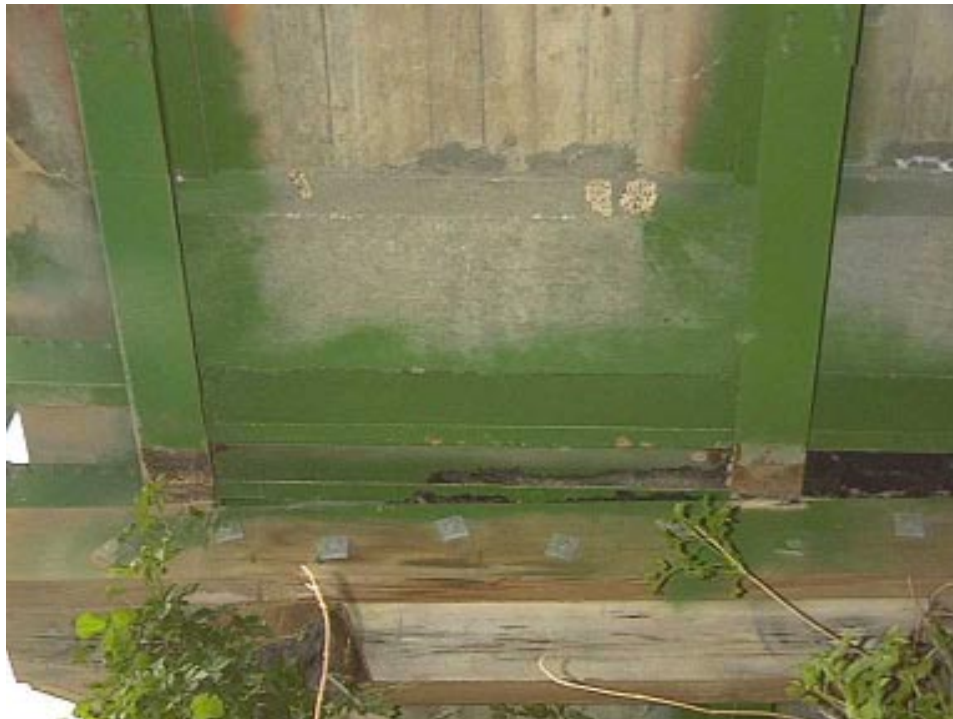
UNDERSIDE OF BRIDGE DECK AND TIMBER CAPBEAM
