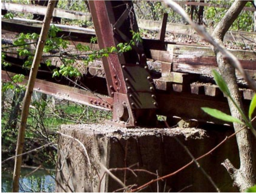
ENDPOST AND BEARING OF STEEL TRUSS
