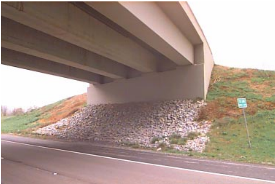
CONCRETE BRIDGE ABUTMENT
