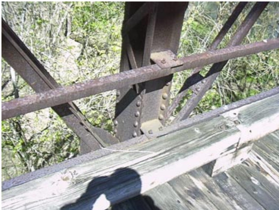
STEEL TRUSS CONNECTION
