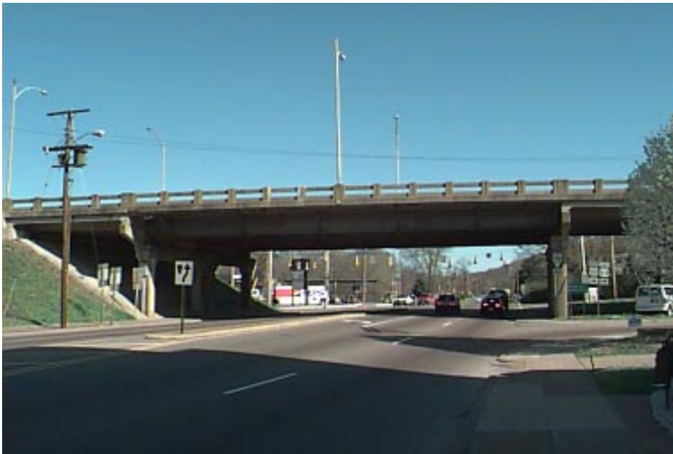
ELEVATION VIEW OF ROADWAY UNDERPASS
