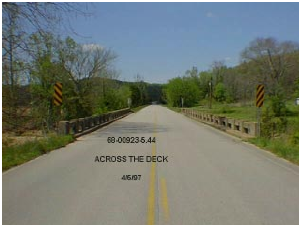
VIEW ACROSS BRIDGE DECK
