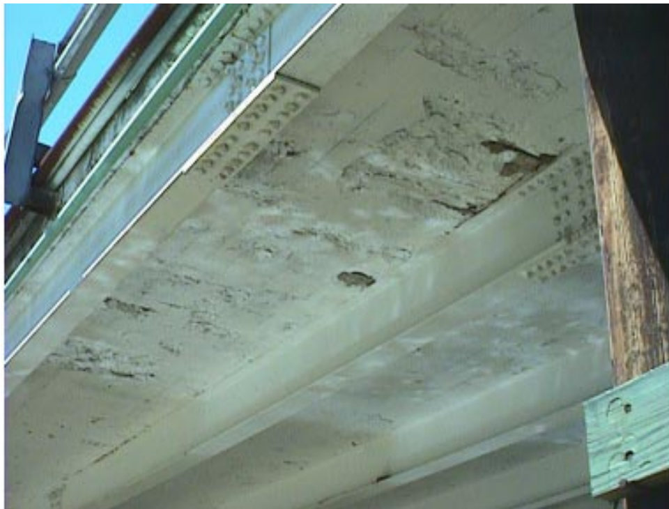
UNDERSIDE OF STEEL BEAM SPAN
