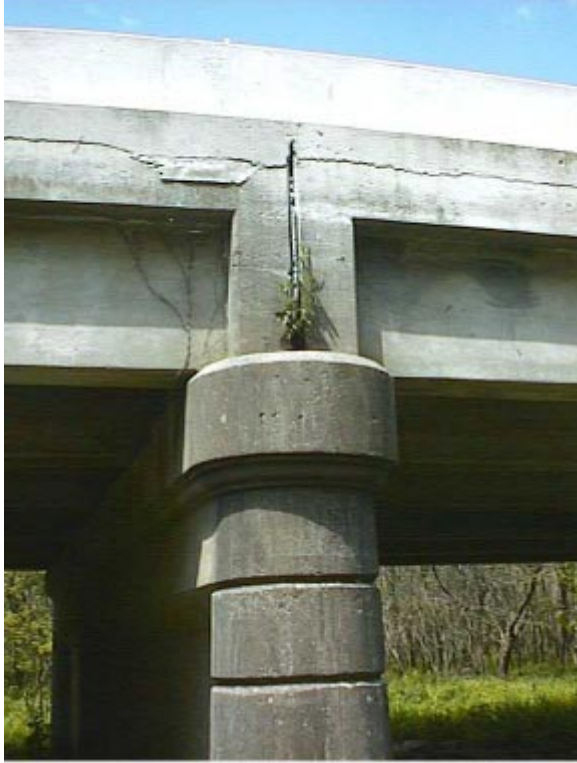
CONCRETE BRIDGE PIER
