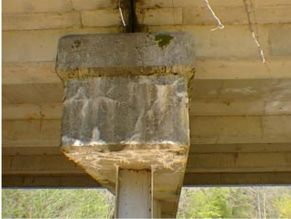
END OF BENT CAP
