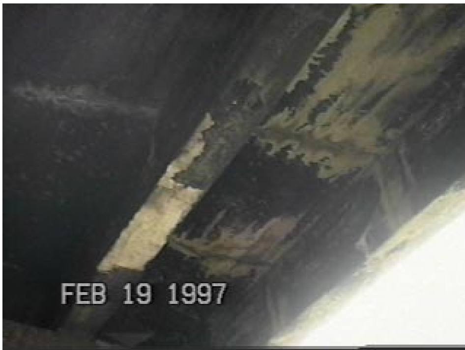
UNDERSIDE OF BRIDGE DECK
